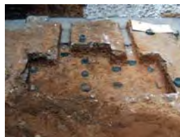
DSCF2058 Final Cala 1 i riostres Nord
