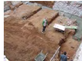
DSCF2049 Vista general riostres Nord
