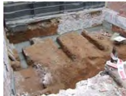
DSCF2048 Vista general riostres Nord
