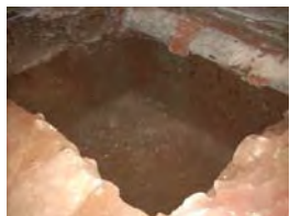
DSCN2623 Vista general final
